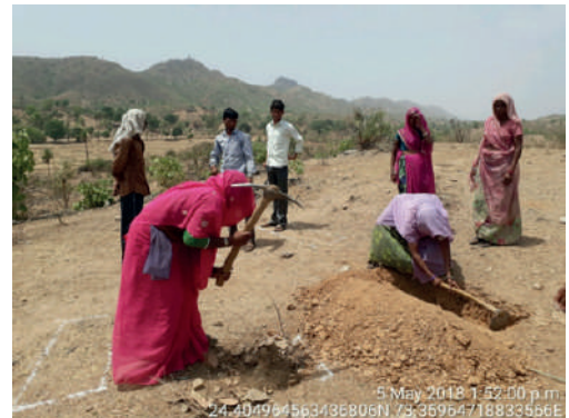
Pit digging at Kakarmala village in Jhadol block
