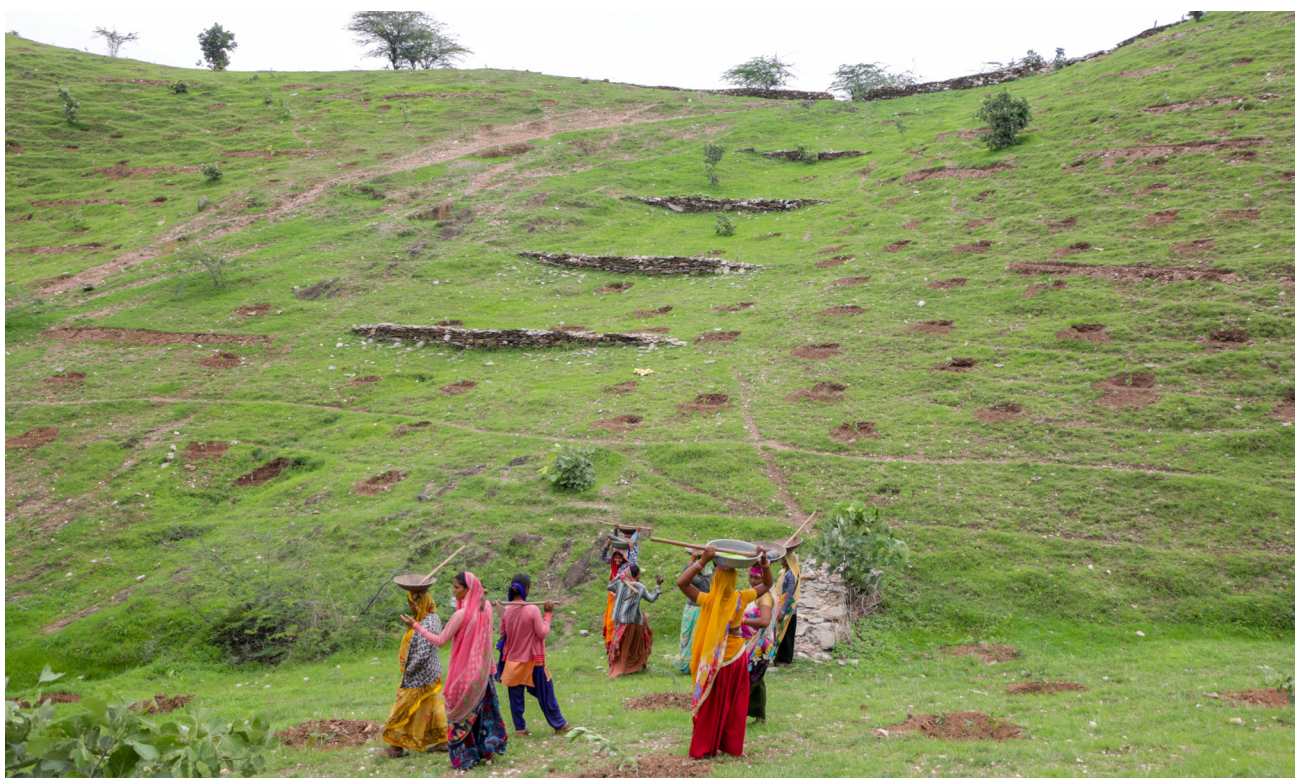
Newly constructed gully plugs on a pasture land in Kherwara to restrict rain water run-off
