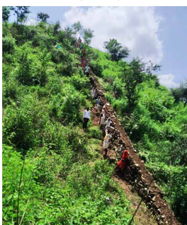
Loose-stone protection of new site
