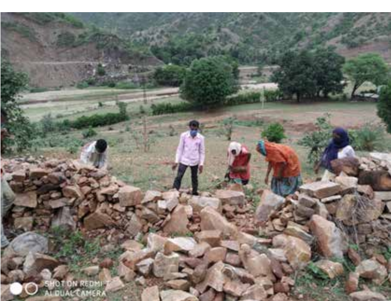
Loose-stone protection wall construction
