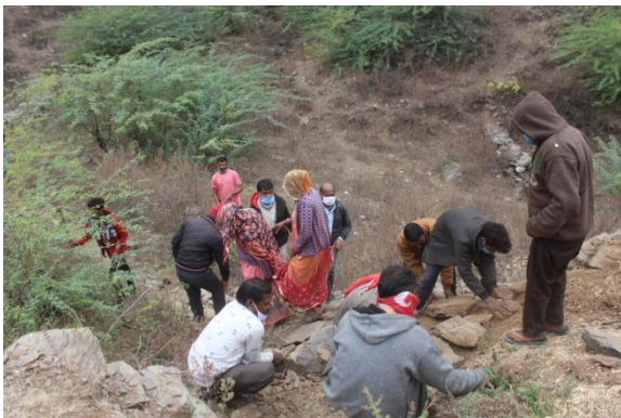
Loose-stone protection wall repairing- Shramdaan
