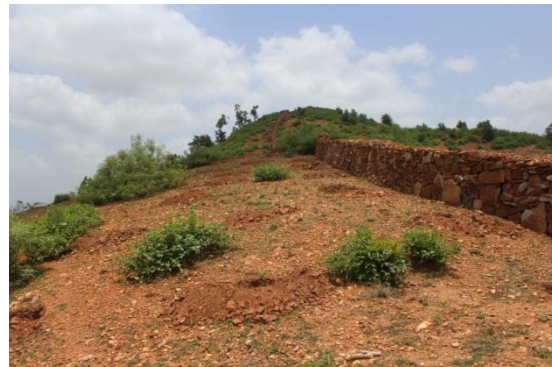
Completed loose-stone protection wall
