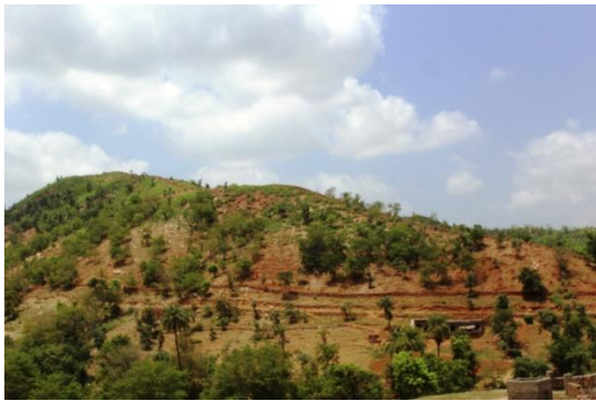
Completed loose-stone protection wall
