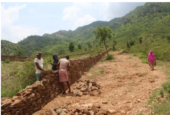
Loose-stone protection wall
