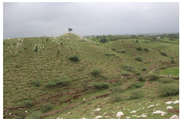
Completed loose-stone protection wall
