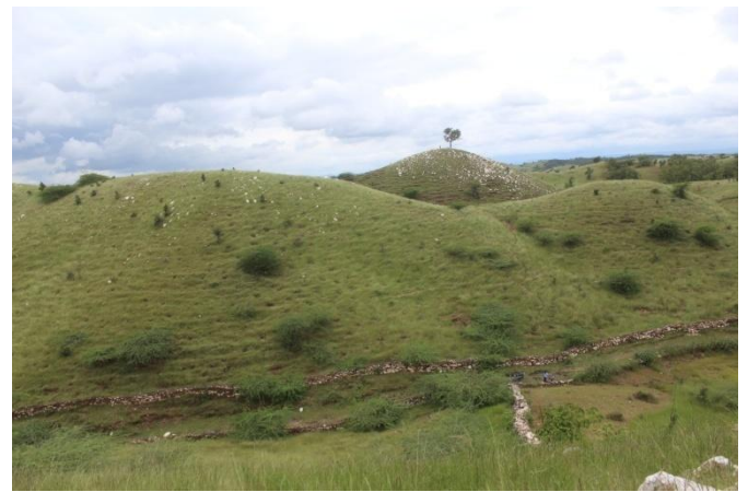
Maintained loose-stone protection wall
