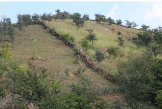
Maintained loose-stone protection wall
