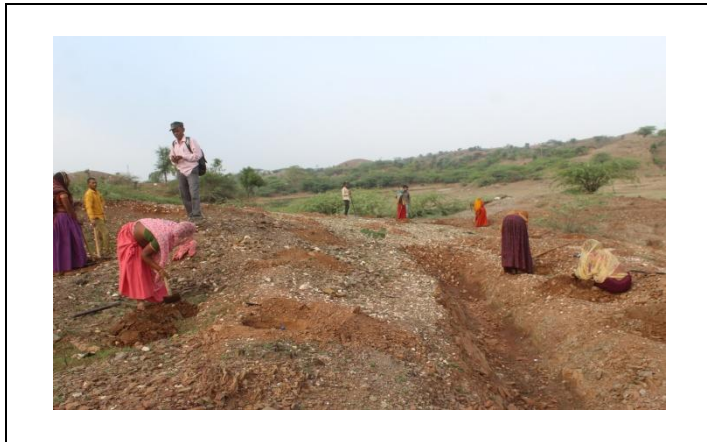
On-going pit digging work
