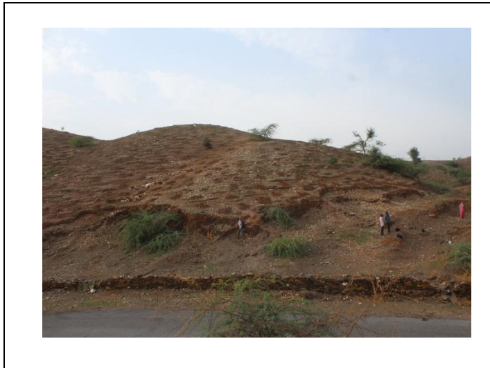
Site completed for plantation
