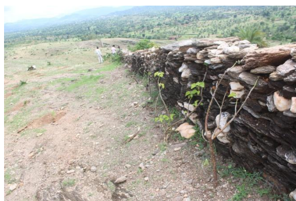
Completed loose-stone protection wall
