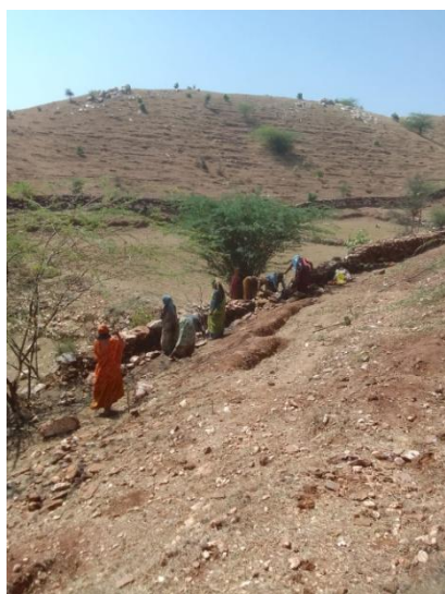
Ongoing physical activities – Loose stone protection wall
