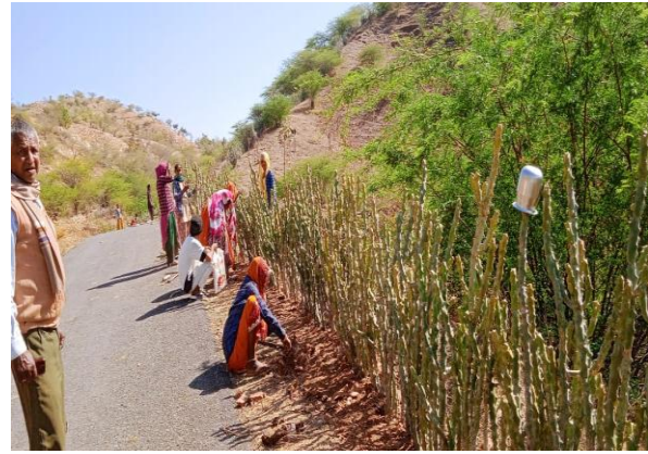
On-going thor bio-fencing work at the site
