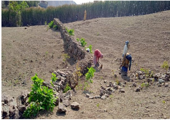
On-going loose-stone protection wall
