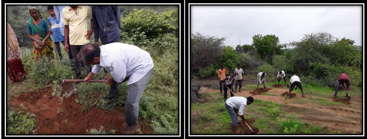
PIT-DIGGING AND CLEARING ACTIVITY FOR SITE PREPARATION
