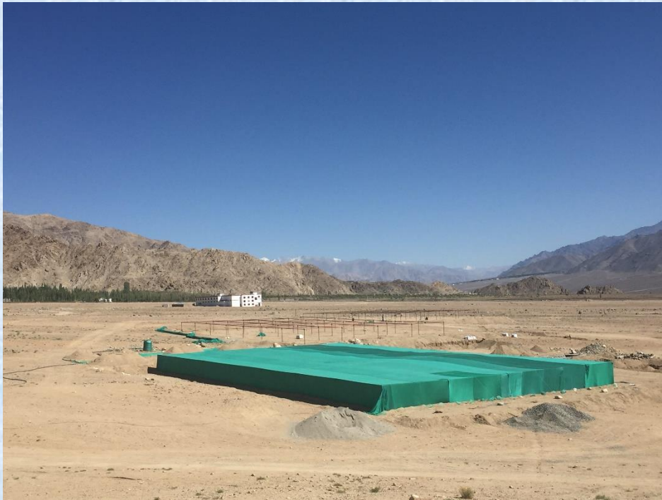
Figure 7. Nursery 1 shade net installed and Nursery 2 & 3 frames erected. Photo from September 12 th .
