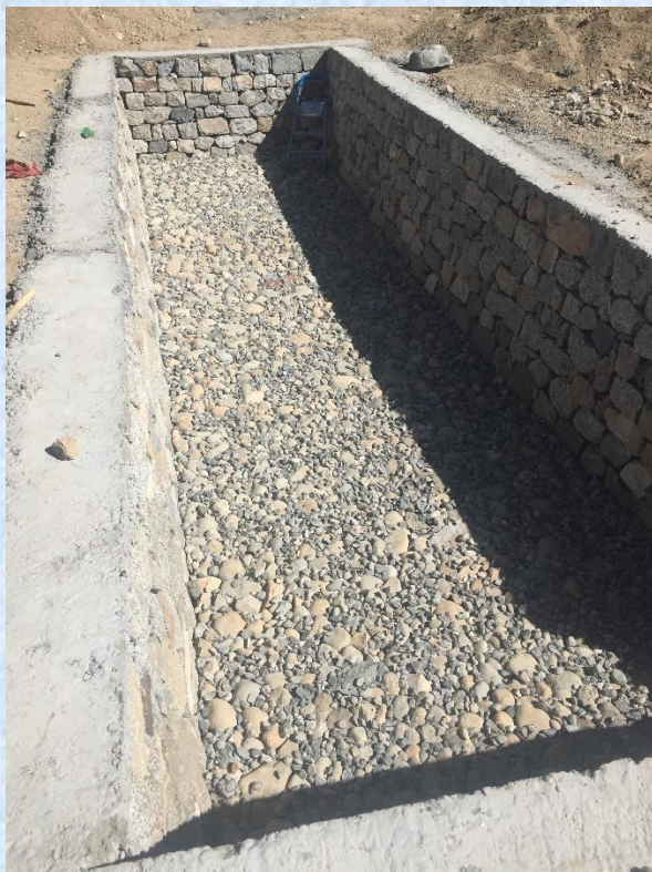
Figures 8 & 9. Stone work of the polytrench and then covered with plastic for germinating seeds, base layer enhances soil warmth. Photos from September 23 rd & 29 th .
