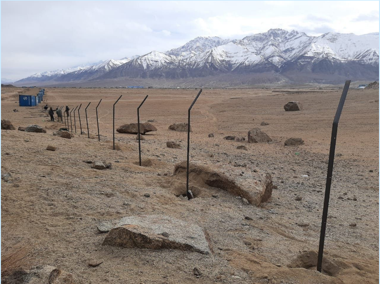
Figure 11. Boundary fence under construction.
