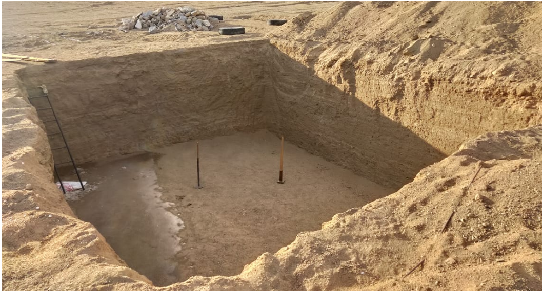
Figure 9: Excavation Work for Root Cellar
