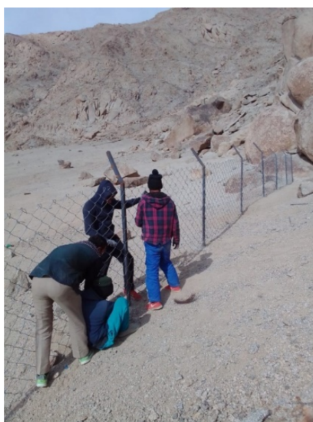
Figure 6: HIAL Boundary Fencing work continues
