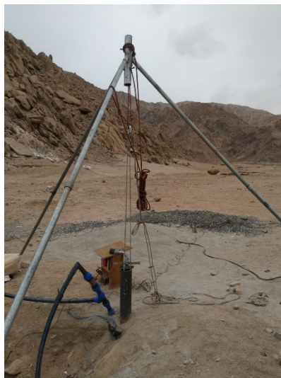
Figure 8: Borewell Repair work in Progress
