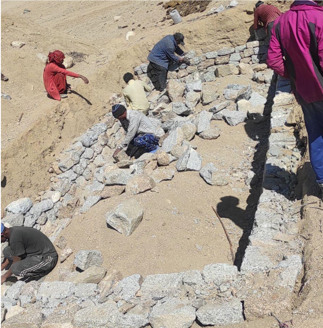
Fig 10: Trench construction under process
