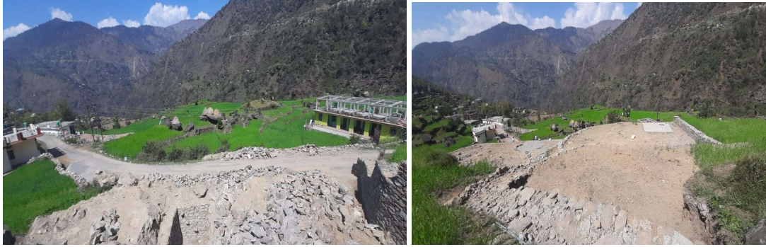
Ground Work under MNREGA undertaken at Makku Math Homestay sites
