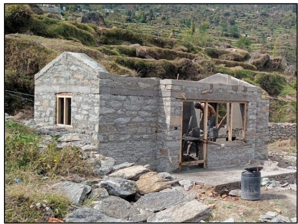
Plaster completed in Makku Homestays
