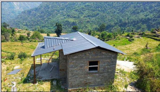
HOMESTAY ROOF IN MAKKUMATH
