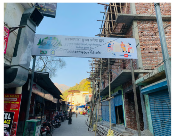
Big Entrance Board Installation
