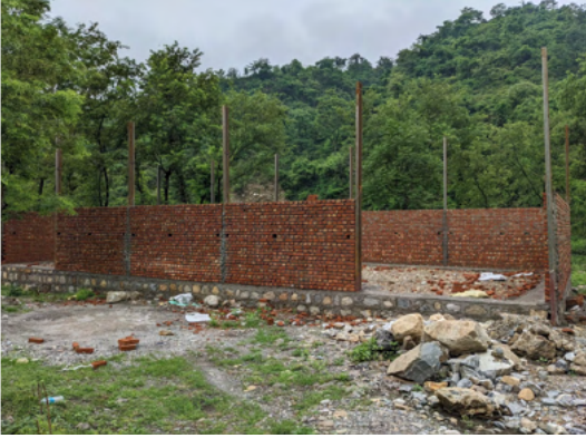
MRF Construction at Bandawali
