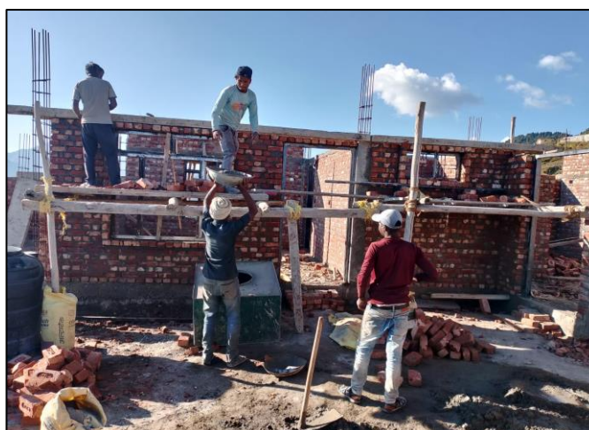
Building work of the community café in the Jadipani Cluster
