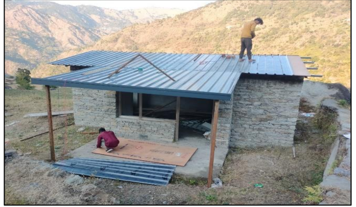
Roofing work of all six homestay completed in Makkumath
