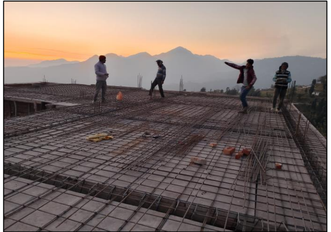
Roof construction of the community café building in Jadipani
