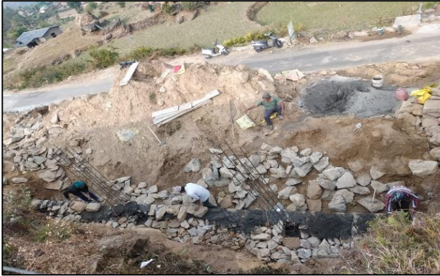
Construction work of seventh homestay restarted in Makkumath village
