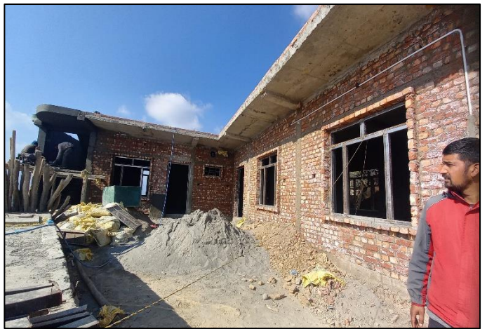
Community café construction work done, interior work to start in Jadipani
