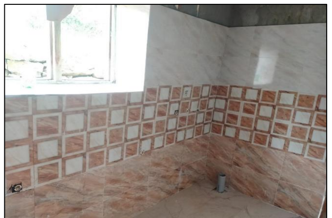
Bath and electric fittings work completed in six homestays in Makkumath
