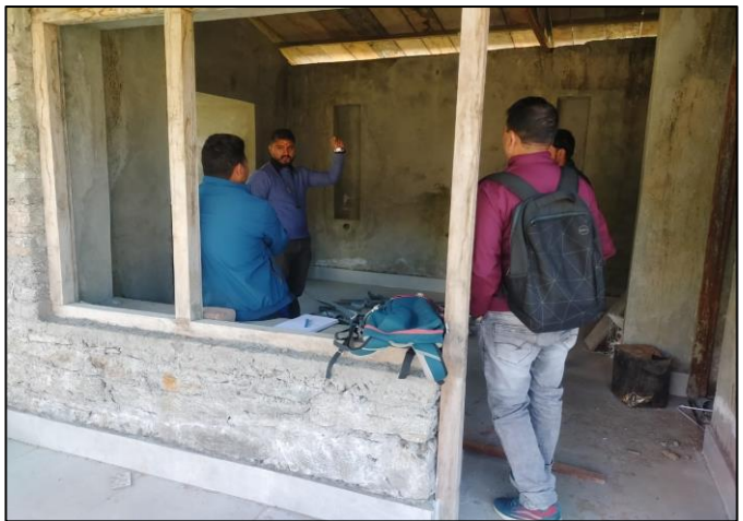
Interior development work of homestays started in the Makkumath cluster
