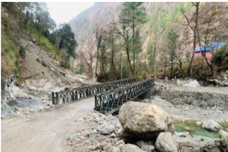
Figure 8: Second Bailey Bridge in Nivli Village, Sainj Valley
