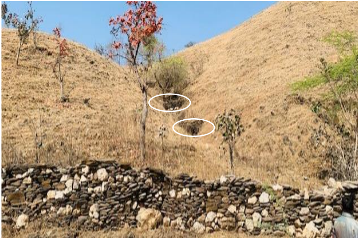
Figure 31: Check dams in the pastureland, along with stone boundary wall
