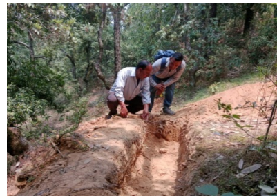
Construction of Contour Trench
