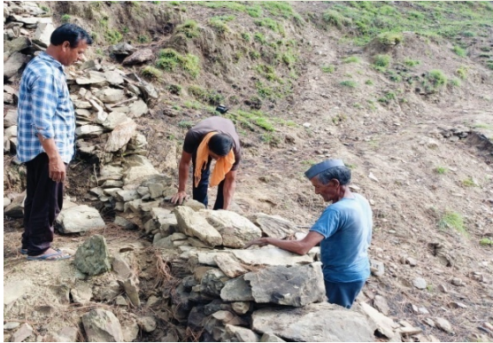
Repairing of Protection Wall in the Van Panchayat
