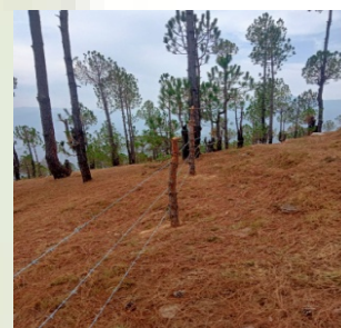
Installation of Barbed Wire Fencing
