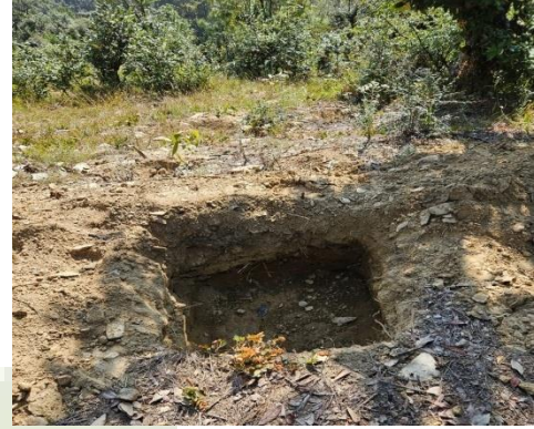
Percolation Pit in Kaltani
