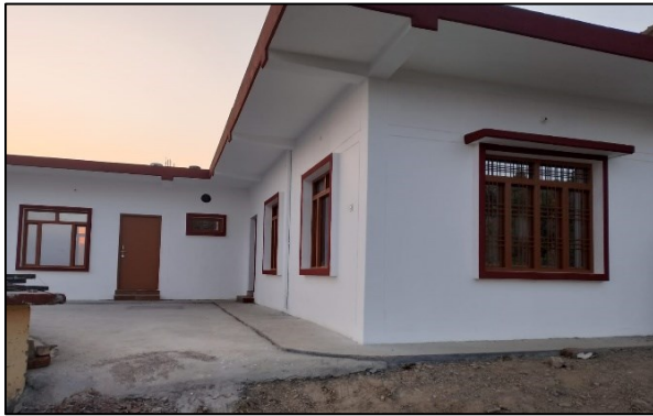
Community Café building completed
